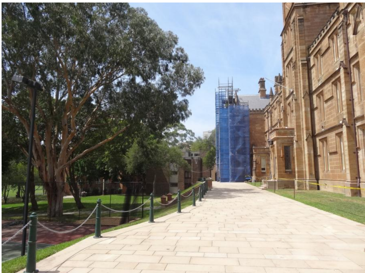
Figure 5: Looking south along the Main building forecourt
