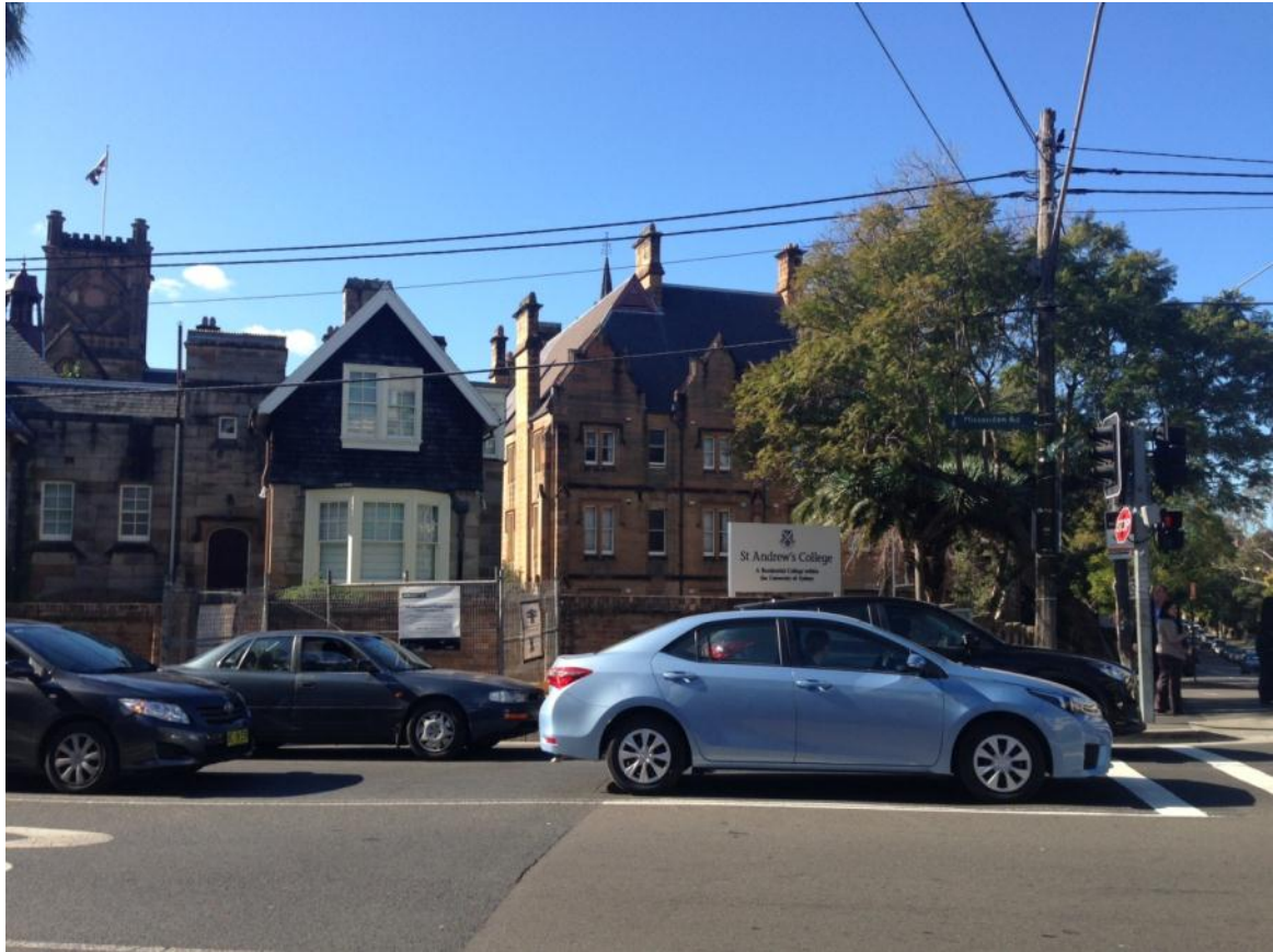
Figure 8: View of Main building Sulman and Vaucluse Wings from Missenden Road looking east
